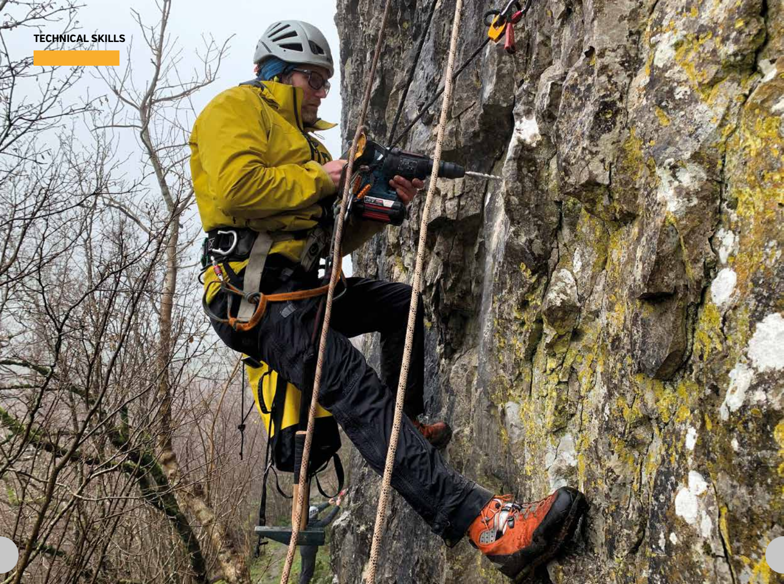
ABOVE BMG member Adrian Nelhams replacing some 1991-vintage bolts at Scout Scar on a CPD workshop.
